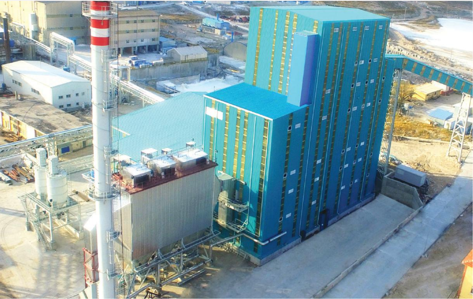
ETİ MADEN TESİSLERİ / KIRKA – ESKİŞEHİR 75 Ton/h 45 Barg 455°C
